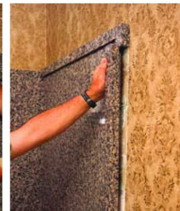
3 Cover the StoneVic trim on the exposed edge profiles.
