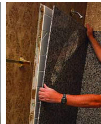
2 Gule the panel directly to the existing wall surface.
