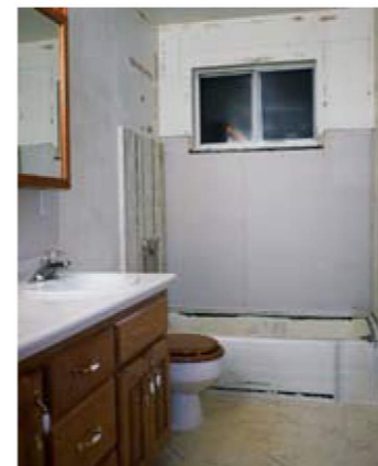
1 Clean the existing surface.
